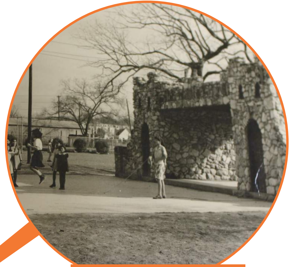
Restored stone work
